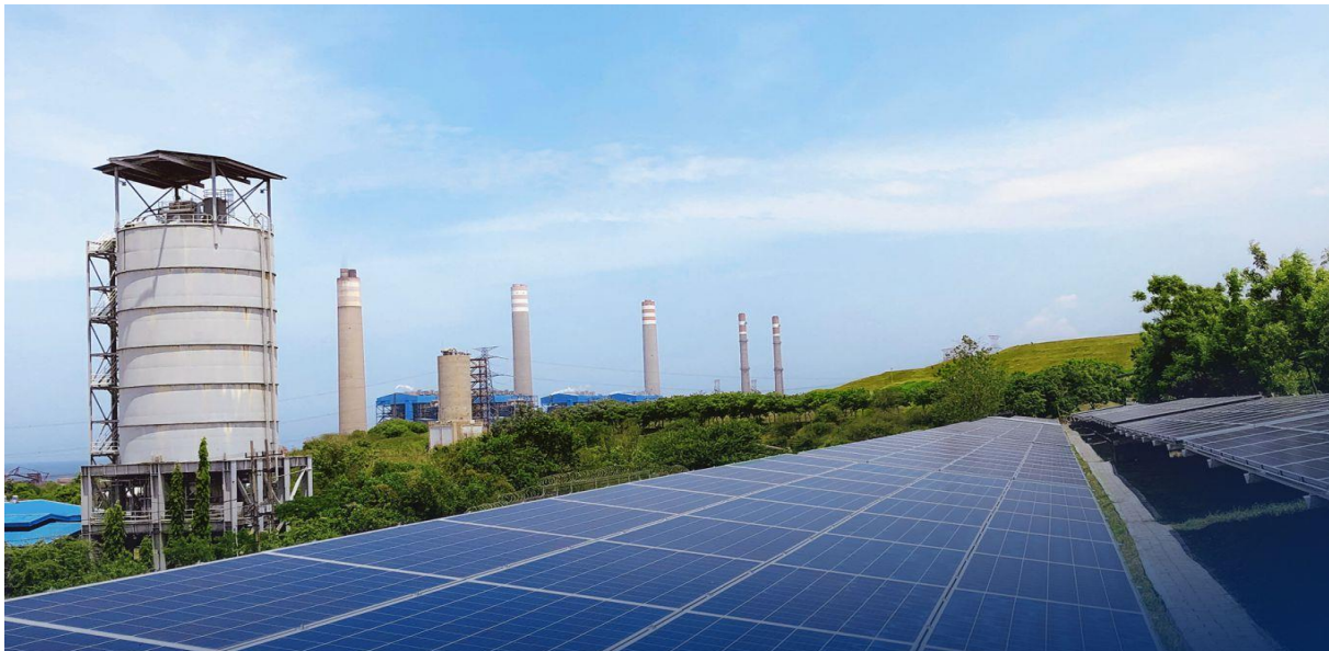
SOLAR PV PROJECT PAITON ENERGY
